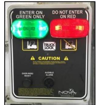
to get an outbound pallet count. Prior to entering the trailer, the lead failed to verify a green checklist was present or investigate the red/green flashing lights. When he finished his count, the lead stepped back out of the trailer and onto the dock plate. The trailer was pulled away from the dock door by a third-party carrier. This action caused the dock plate to drop and the lead to tumble backwards out of the door and onto the pavement.
